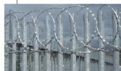
At the upper part of palisade fencing
