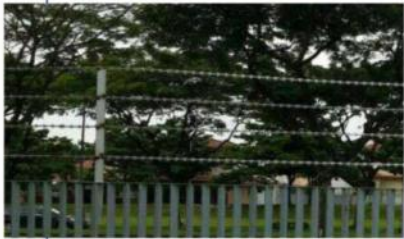
For road perimeter protection
