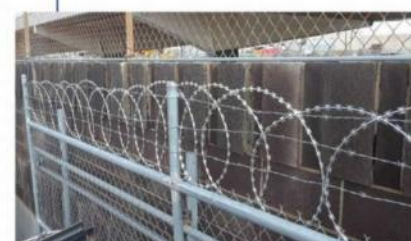
At the top of fence gate
