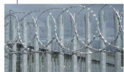
At the upper part of palisade fencing
