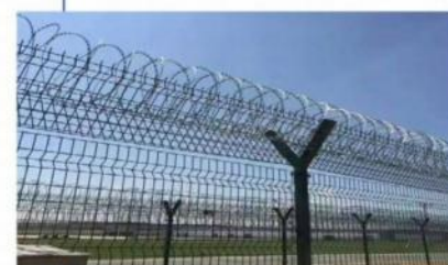
For expressway protection
